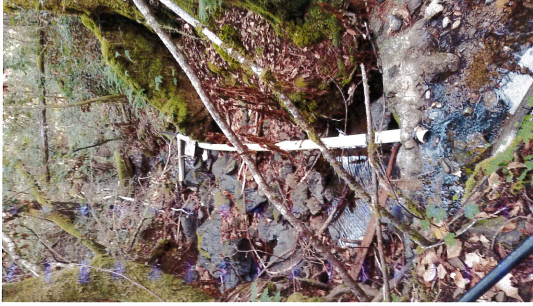
Figure 6. A020134-02: Downstream of present POD Unnamed stream, tributary to Dutch Bill Creek December 29, 2017
